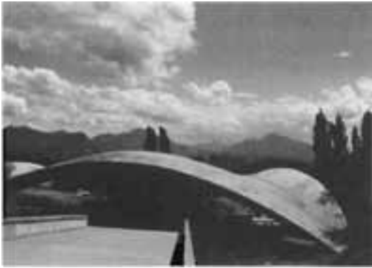
Fig. 1-7 Spherical shell in Lausanne, Switzerland. Upwardly curved edges provide stiffening for the central dome.
