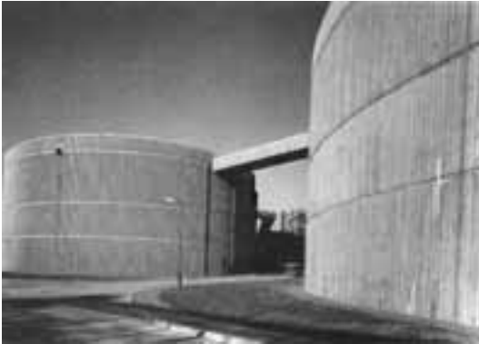
Fig. 1-11 Circular concrete tanks used as a part of the wastewater purification facility at Howden, England (Northumbrian Water Authority with Luder and Jones, Architects).
