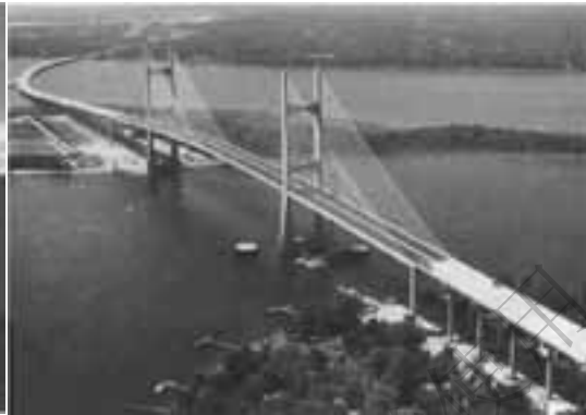
Fig. 1-8 Napoleon Bonaparte Broward Bridge, with a 1300 ft center span at Dame Point, Jacksonville, Florida (HNTB Corporation, Kansas City, Missouri).
