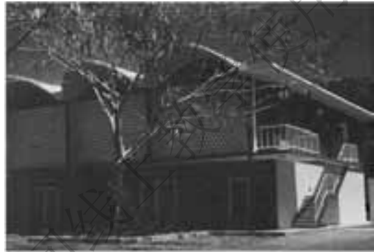
Fig. 1-6 Cylindrical shell roof providing column-free interior space.
