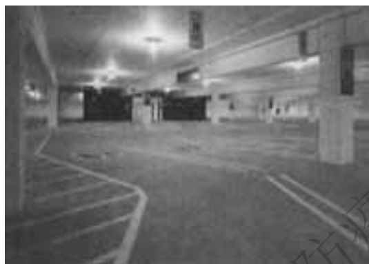
Fig. 1-1 One-way reinforced concrete floor slab with monolithic supporting beams (Portland Cement Association).
