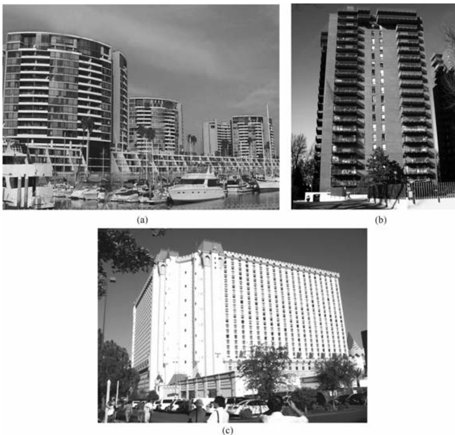
图5 采用配筋砌体承重墙建于美国的高层房屋 (a) Marina Condominiums, Marina, Delaware; (b) Park Lane Tower, Denver, Colorado; (c) Excalibur Hotel, Las Vegas, Nevada
